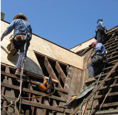
Rey-Crest Roofing employees utilizing proper fall protection
